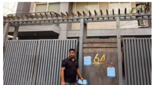
guard outside a sealed property in DLF Phase 3.
